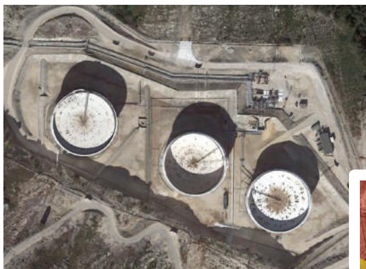
Full storage area retention pond monitored with 5 flames detection cameras
